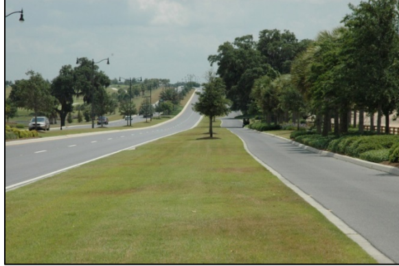
Example of Multi-modal Path along a Right-of-Way
